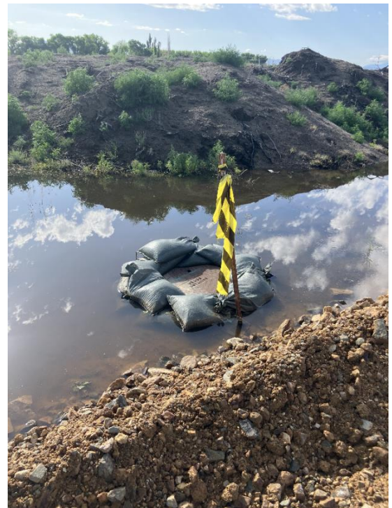
Image of man hole secured from floodwaters during Spring Thaw 2023 (Lyon County Emergency Management)
