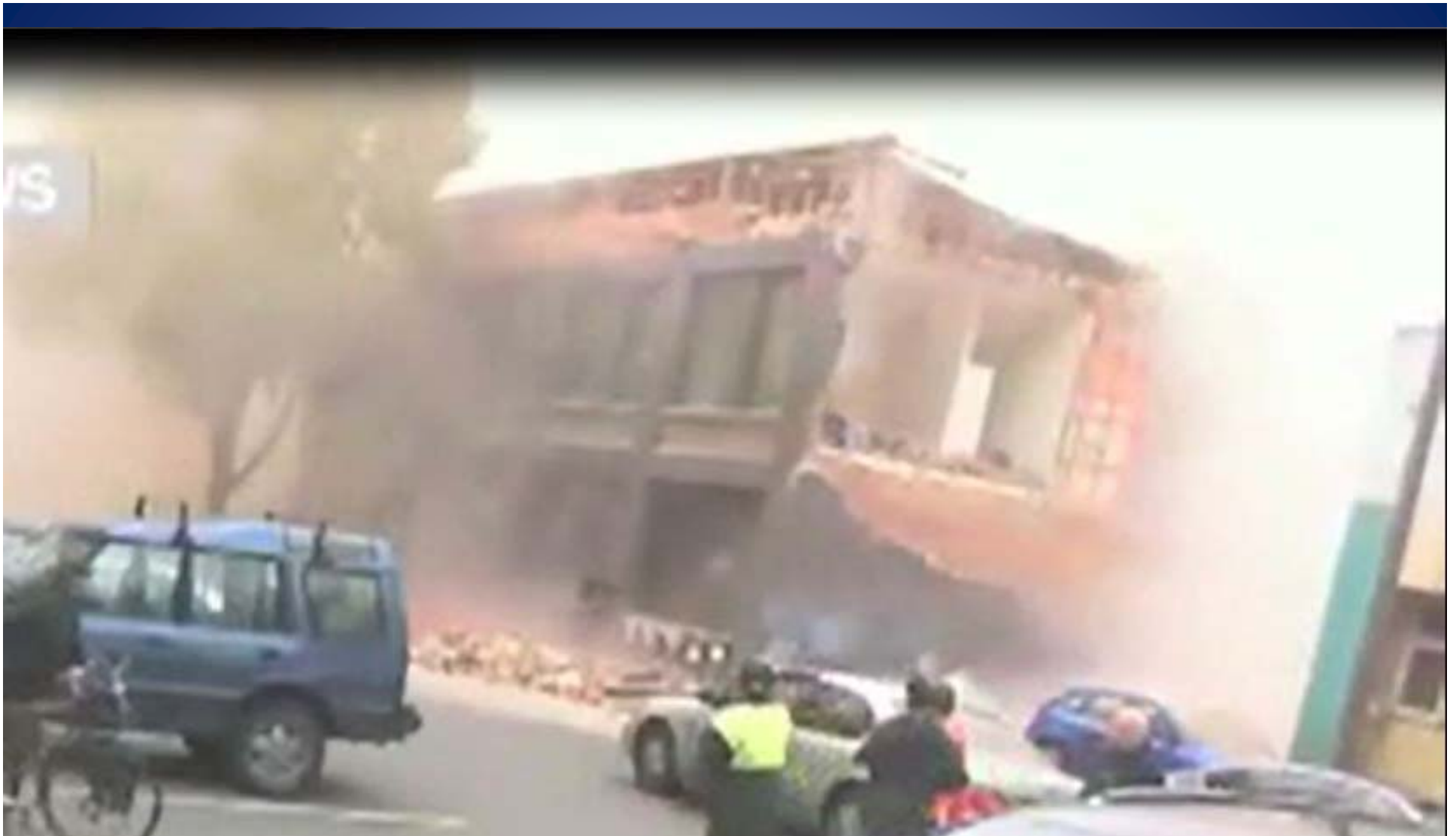
Damaged URM – major failure of right facing wall exposing rooms and Failure of the upper part of the left facing wall. Debris surrounds building.
