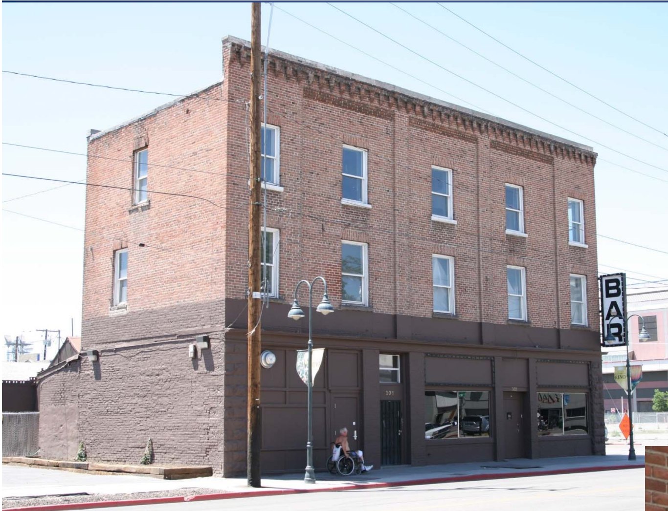
Three-story URM with parapet and some earthquake cracks; occupancy is variable
