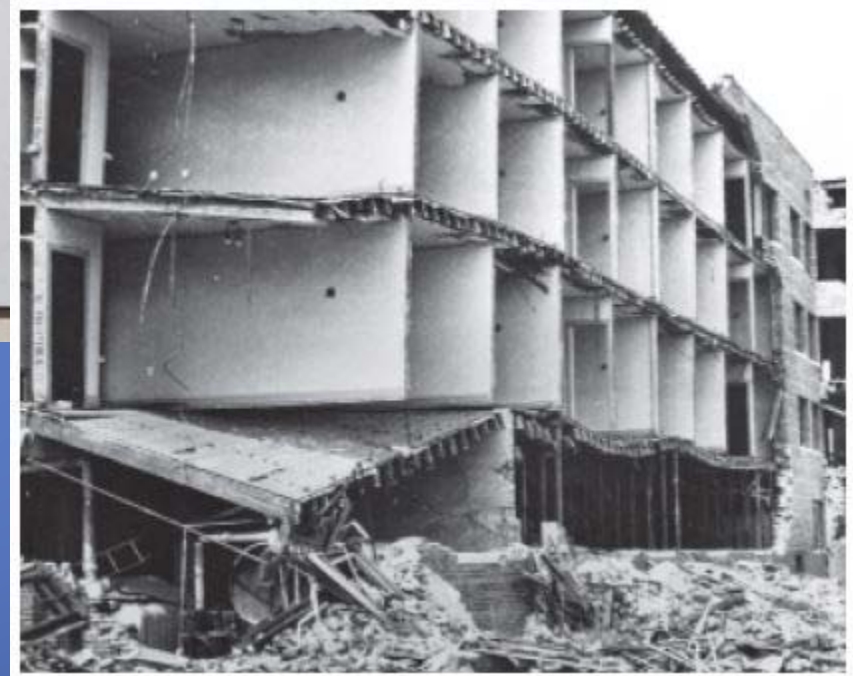
1925 Santa Barbara, California Earthquake Unreinforced Masonry Damage to the Hotel California
