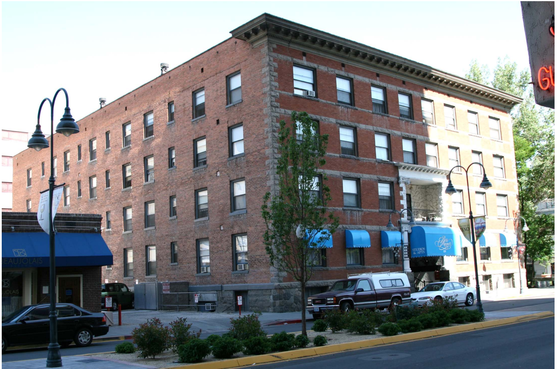
Commercial five-story apartment building; continuous high occupancy
