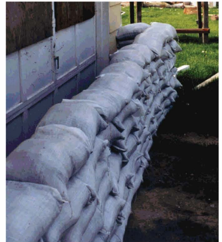
Single stack placement
